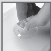
用吸盘打开 Use sucker to open the diffuser
